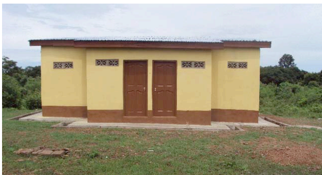
A completed ecological latrine at a school in Prang, a village in Ghana's Brong-Ahfo region
